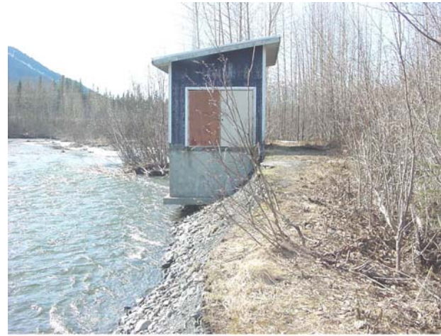
Photo 2: Well head building site relocated, April 2000
