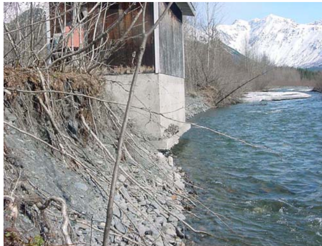
Photo 3: Well head building site relocated, April 2005.
